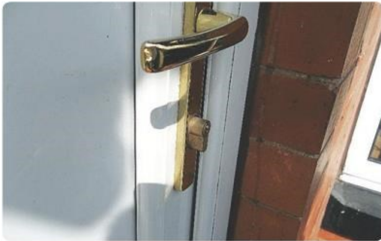
◀ Incorrectly measured lock protruding from the door handle
